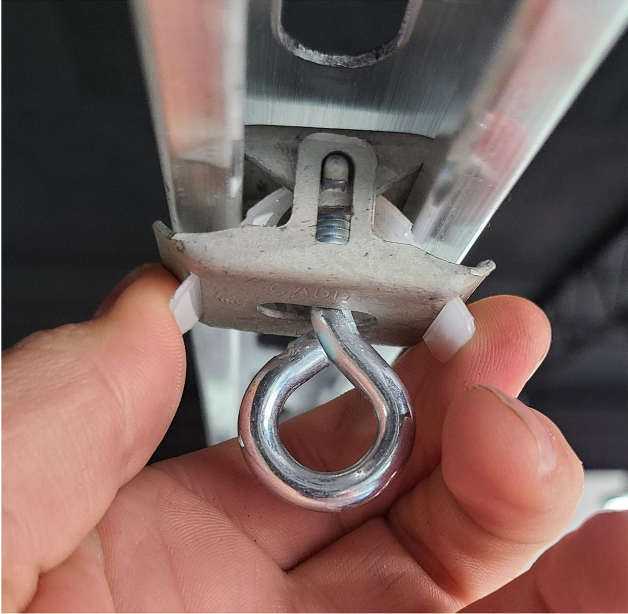
**ONCE THE UNISTRUT IS INSTALLED THE EYE HOOKS CAN EASILY SLIDE INTO PLACE**
